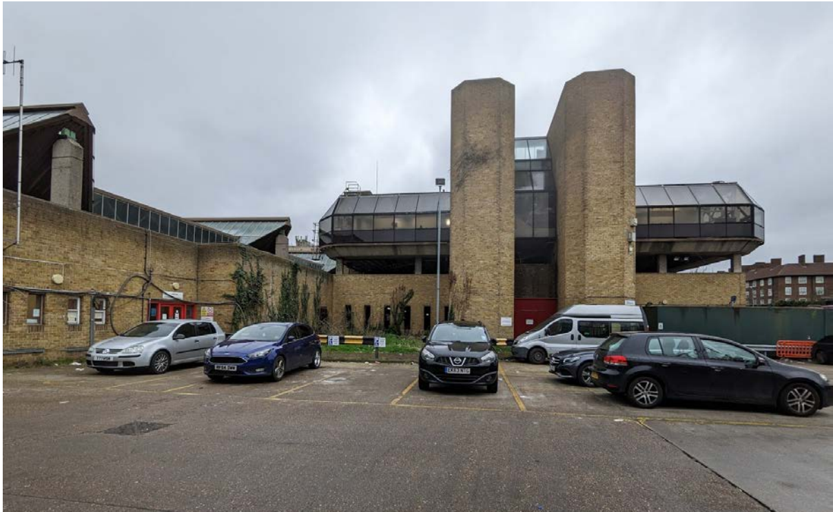
Fig X: Ash Grove bus garage angled stair structures, upper level office and garage roof structure
