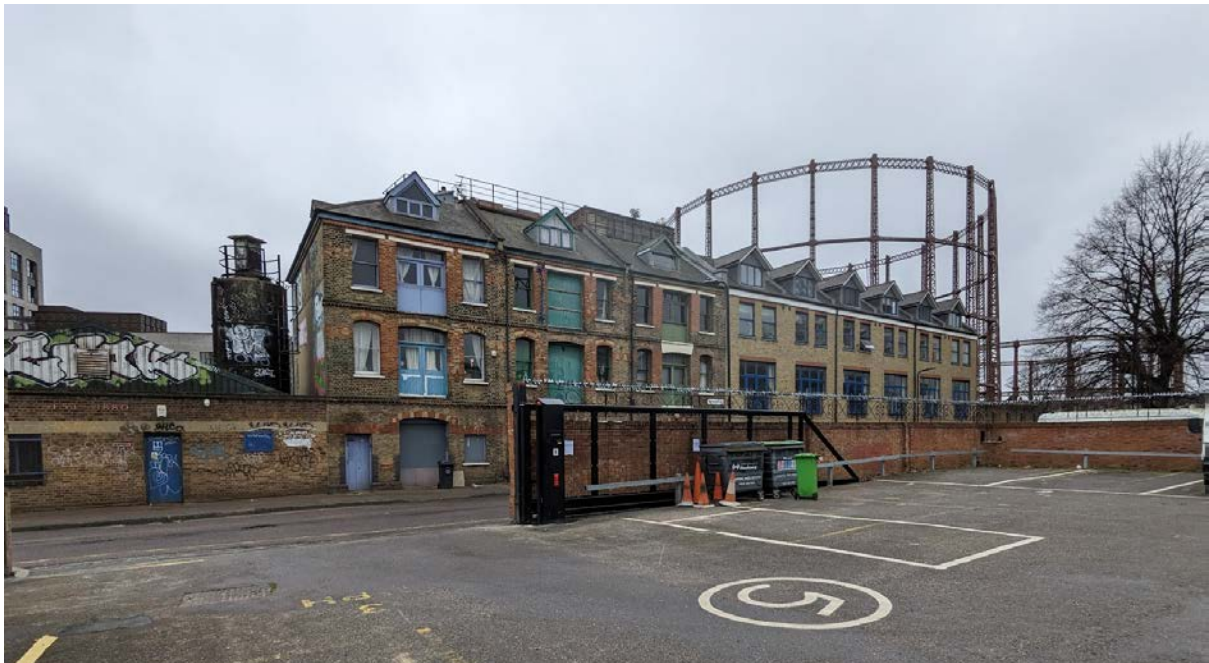
Fig X: Andrews Road warehouses that the canal runs behind
