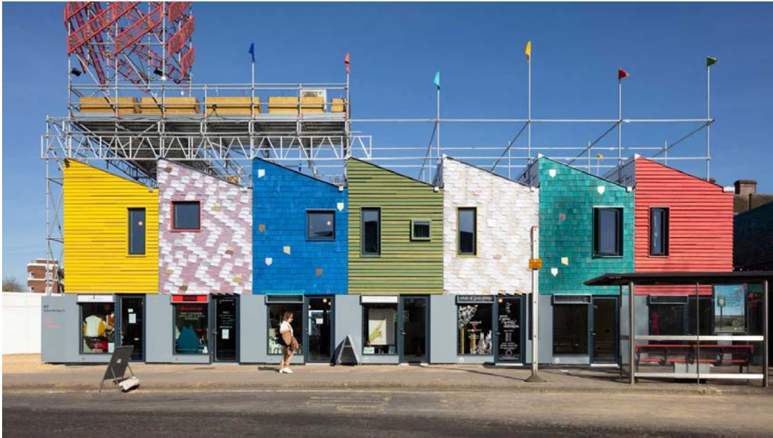
Fig X: Ebury Edge, London can be disassembled, relocated and reassembled multiple times 69
