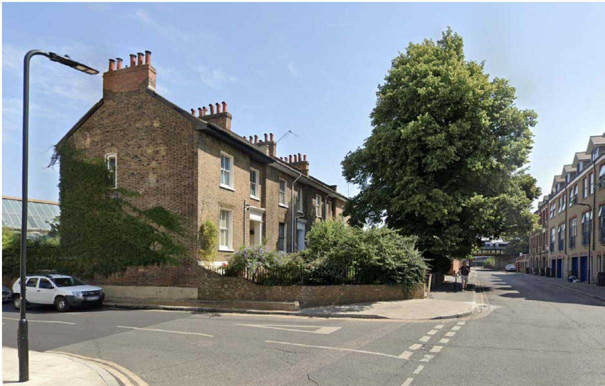
Fig X: Locally listed Victorian terraced houses at 35-38 Andrews Road
