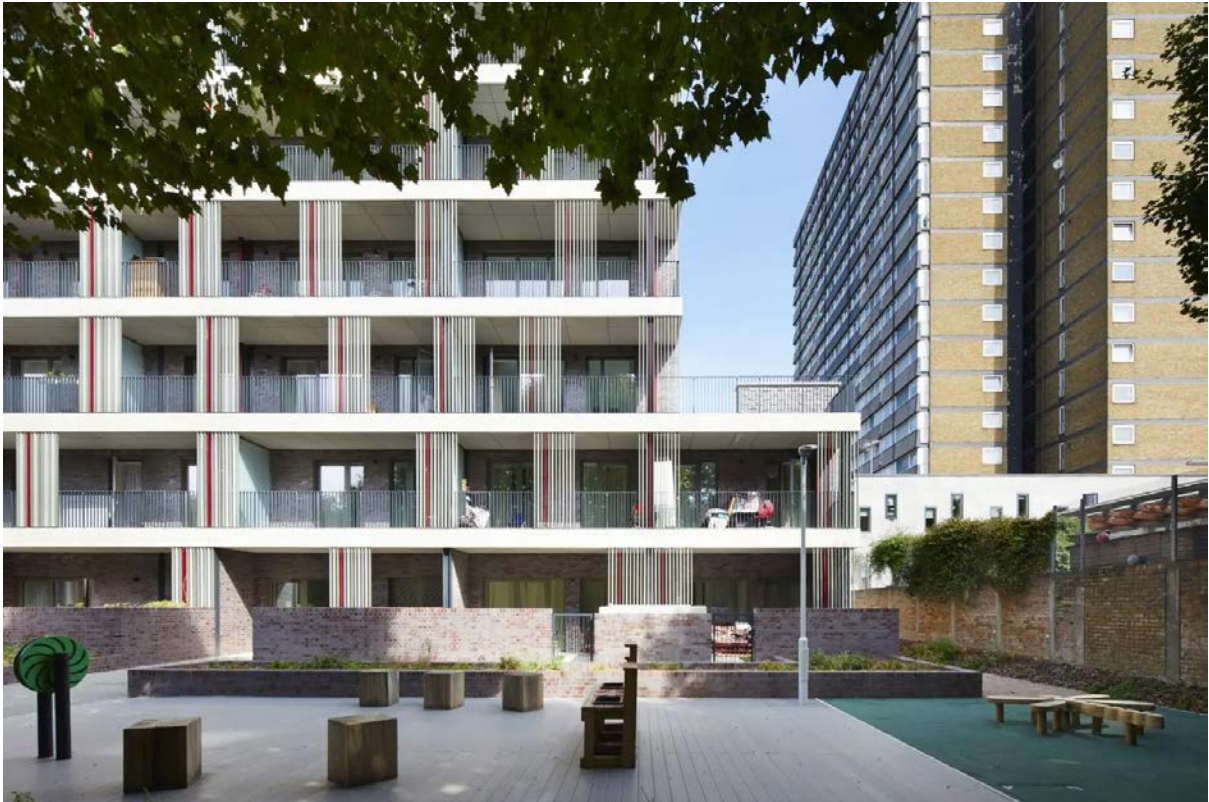
Fig X: Agar Grove by Hawkins Brown is the largest Passivhaus development in the UK, it has a optimised form and the balconies shade the homes from the sun to reduce overheating 64
