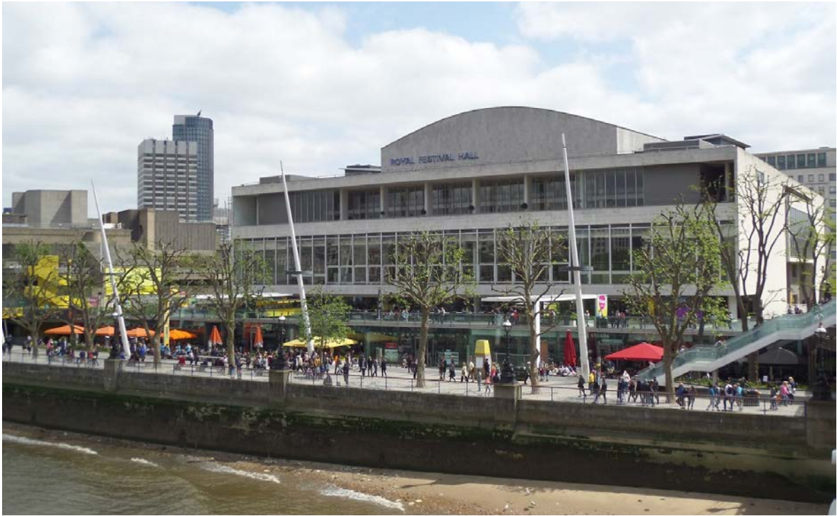
Fig X: access to the upper deck of the South Bank is via the Royal Festival Hall
